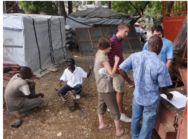
Figure 5. Students worked with local metal fabricators and builders to gain a better understanding of the building practices and construction techniques
